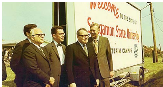
Sangamon State University groundbreaking, June 1970
