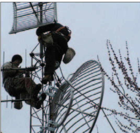
Goin' digital: Workers build the new digital tower for WUIS/WIPA.
