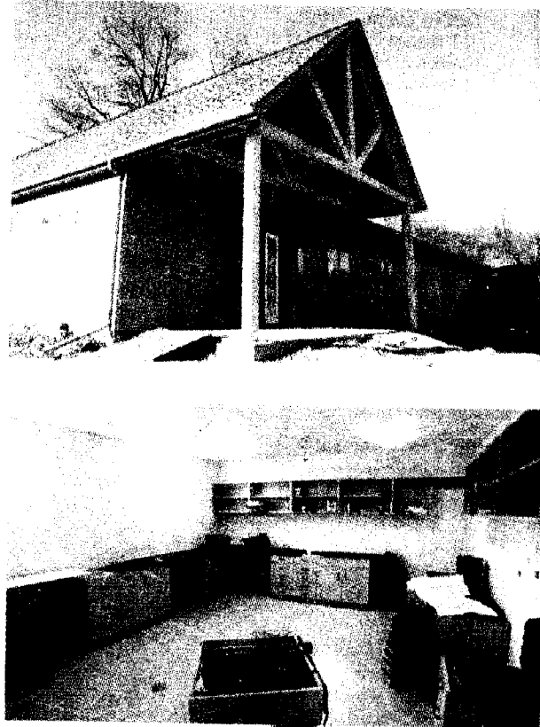
Top: The new University of Illinois at Springfield Emiquon Field Station is nearing completion at The Nature Conservancy's Emiquon Preserve Bottom: Cabinetry is being installed in work areas.
