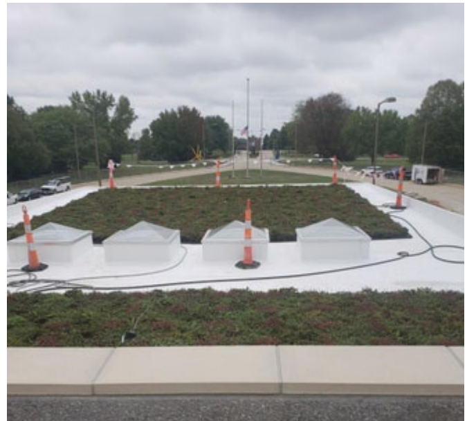
Vegetated roof on the new PAC teardrop entrance
