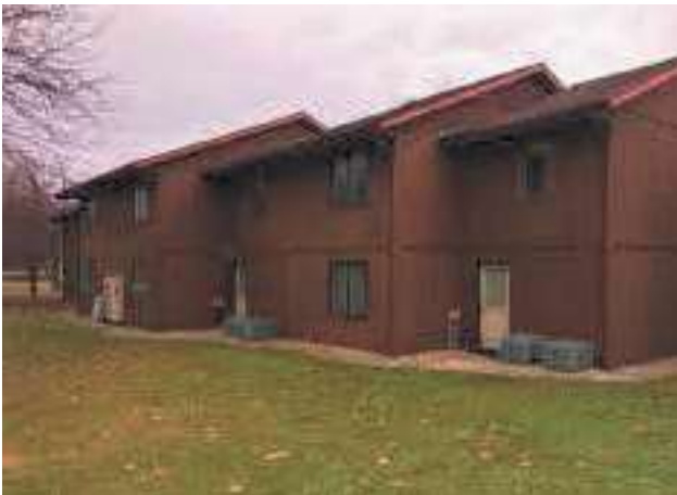
Clover Court Apartments Photos courtesy of Lawrence Group
