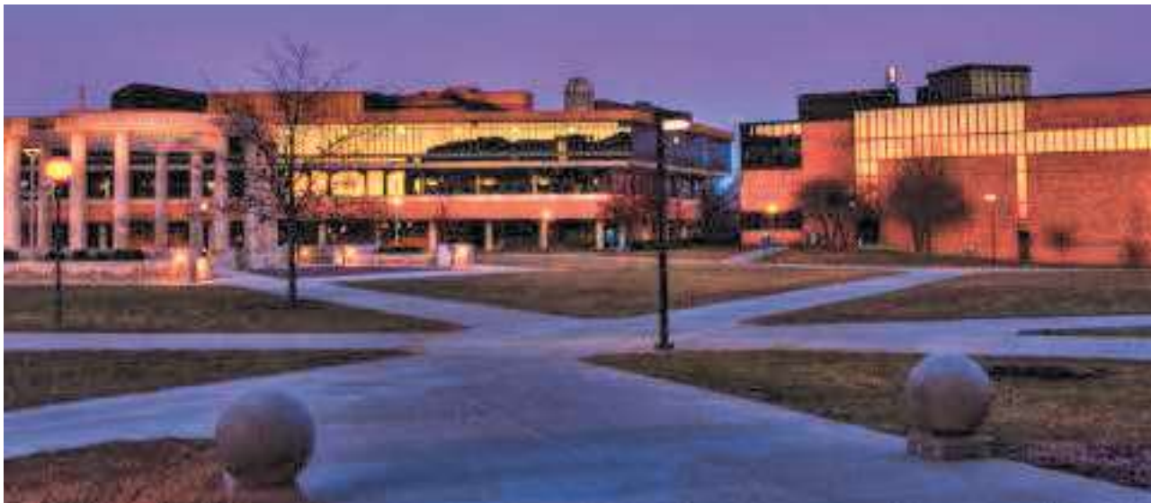
View of Public Affairs Center (PAC) & Brookens Building (BRK) across the Main Quad at dusk. Photo courtesy of UIS.
