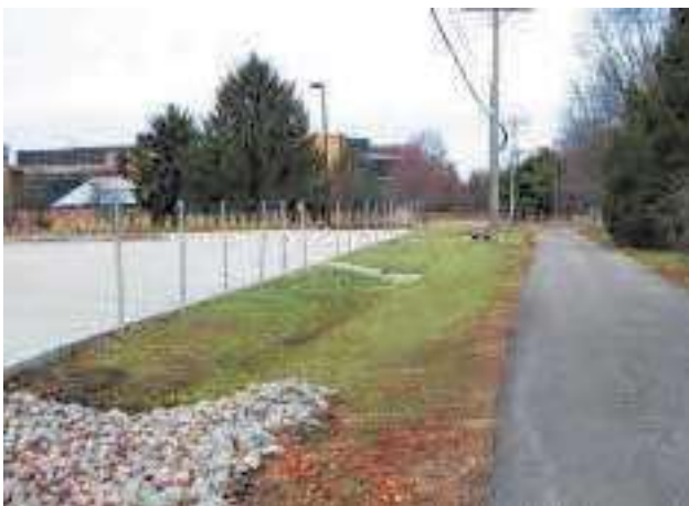
South Campus Drainage Ditch
